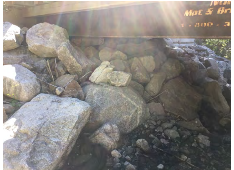
Left Bank Abutment when facing downstream
