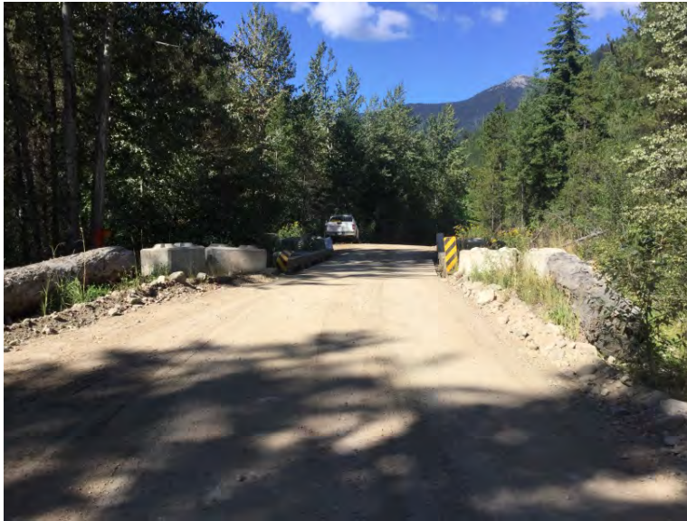
Approach from Left Bank when facing downstream
