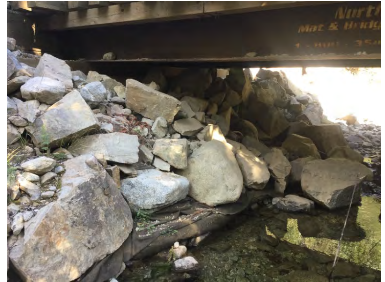
Right Bank Abutment when facing downstream
